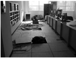
③ DCS Room 제어Cable Pulling
